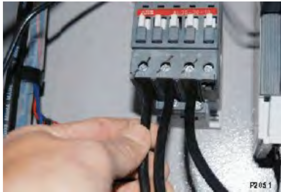
Figure 4-3. Pull-test of cable screw terminal connection
