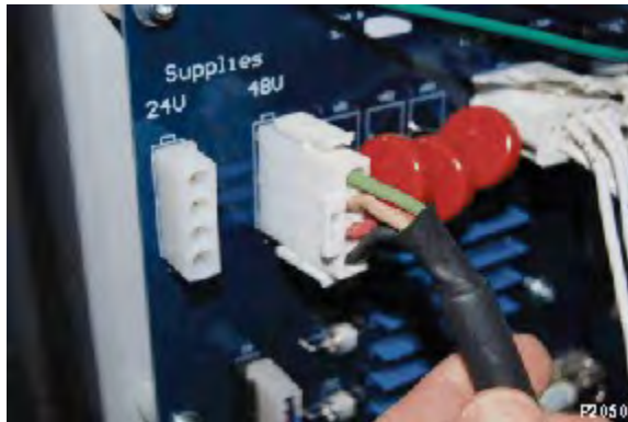
Figure 4-2. Inspection of the cable connections
